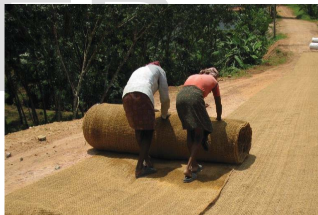
Fig. 4 Coir geotextiles being layed in Attukal Pampadi road on 24.9.2011
