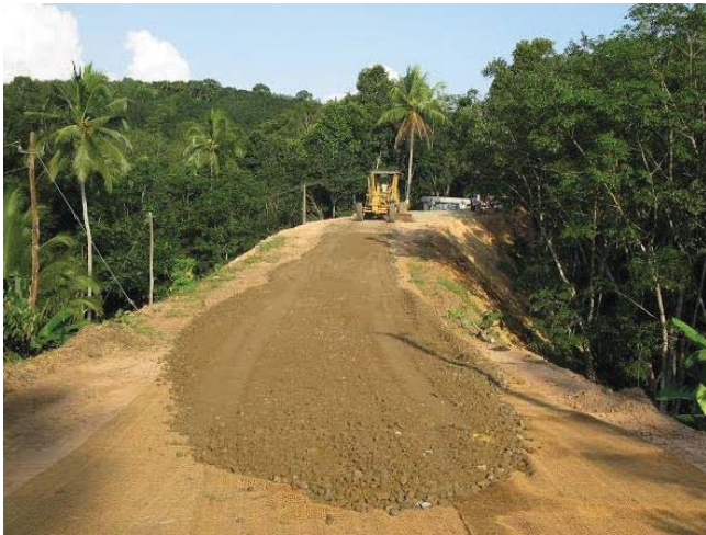
Fig.5 Laying GSB layer over coir geotextiles in Attukal Pambadi road
