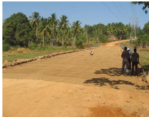
Fig.3 Levelling of road before laying coir geotextiles
